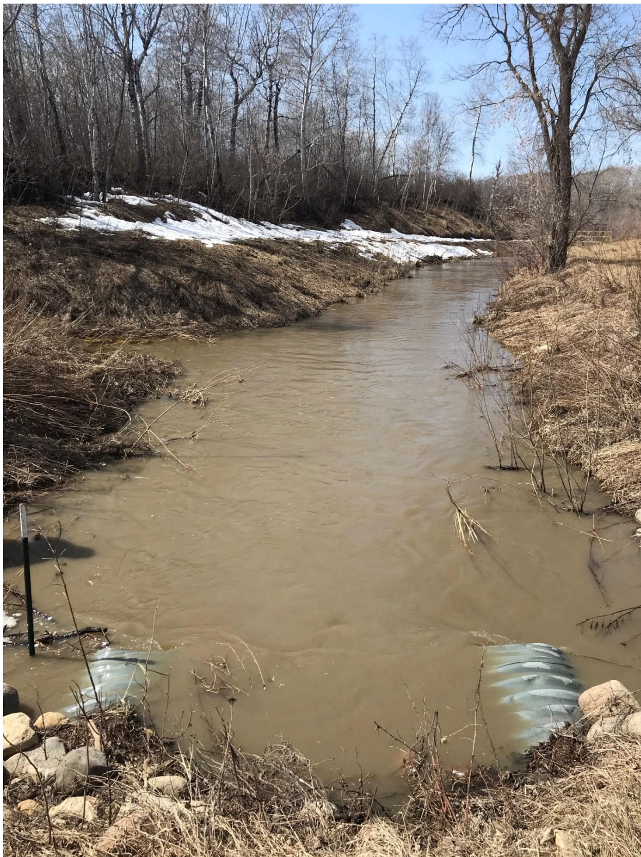
Appendix 8: Culverts visible - a good indication of water levels with velocities tolerable for fish passage ( <1.5\text{m/s} )
