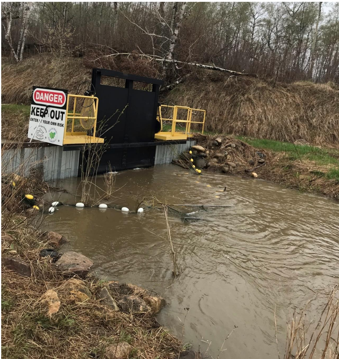
Figure 5: Honoway Fishway Netting Location - May 19 th , 2022
