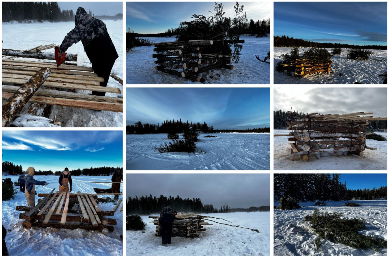
Figure 13: Construction and examples of fish habitat structures - cribs and brush piles
