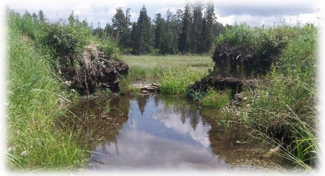
Fig: Blown Dam - North End
